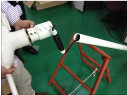
④ Pass the lead wire through the pole.
